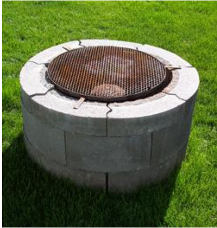
Needs a non-combustible base
