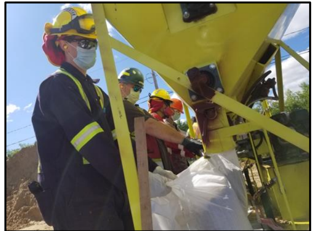
Left: a water-filled berm that was set up to protect a house which was threatened by the high water levels. Right: the sandbagging machine.
