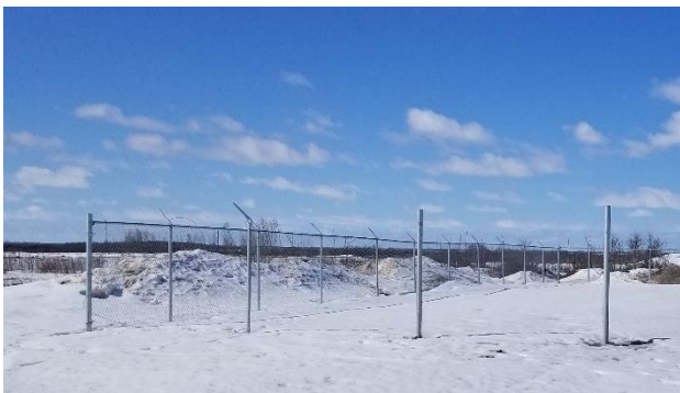
A progress photo of the compound prior to completion
