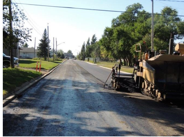
Figure 6: Paving on 6 th Ave W
