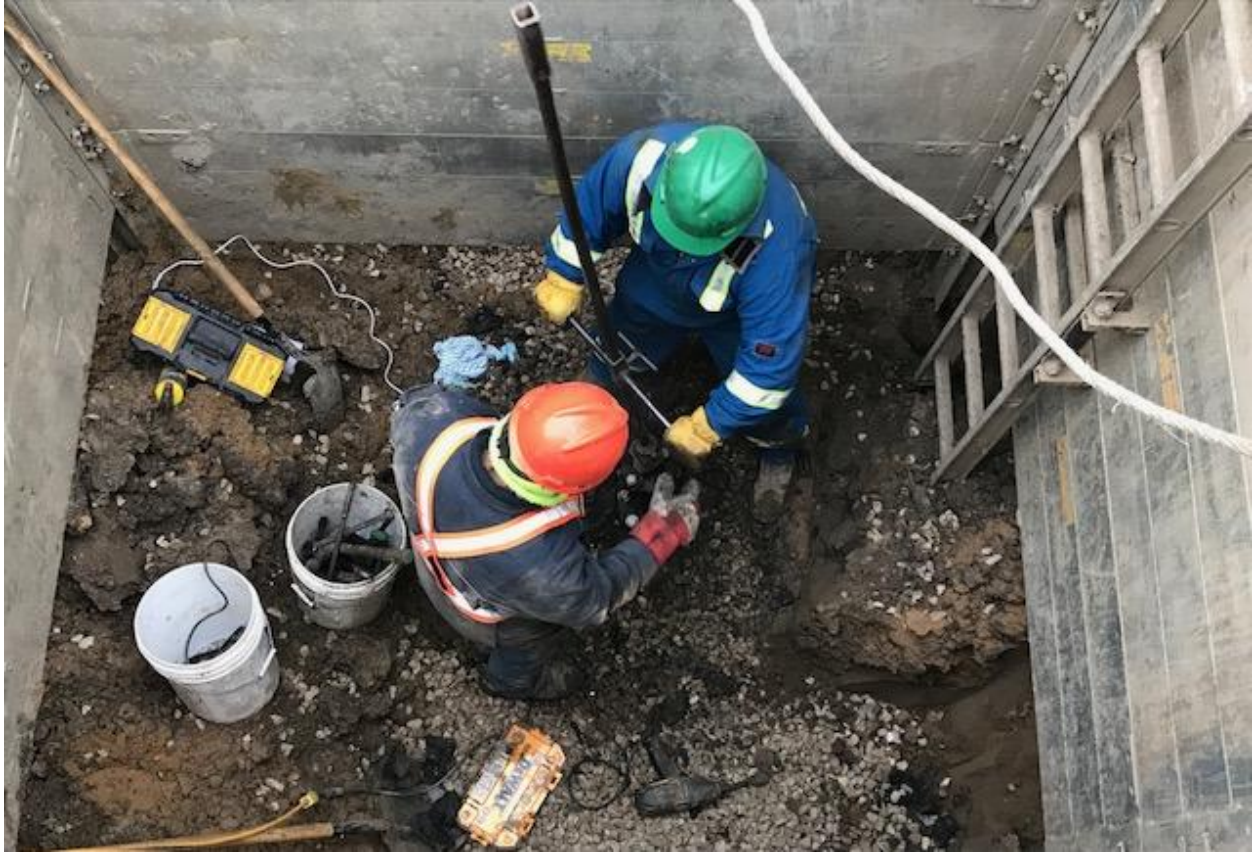
Figure 11: Valve maintenance works
