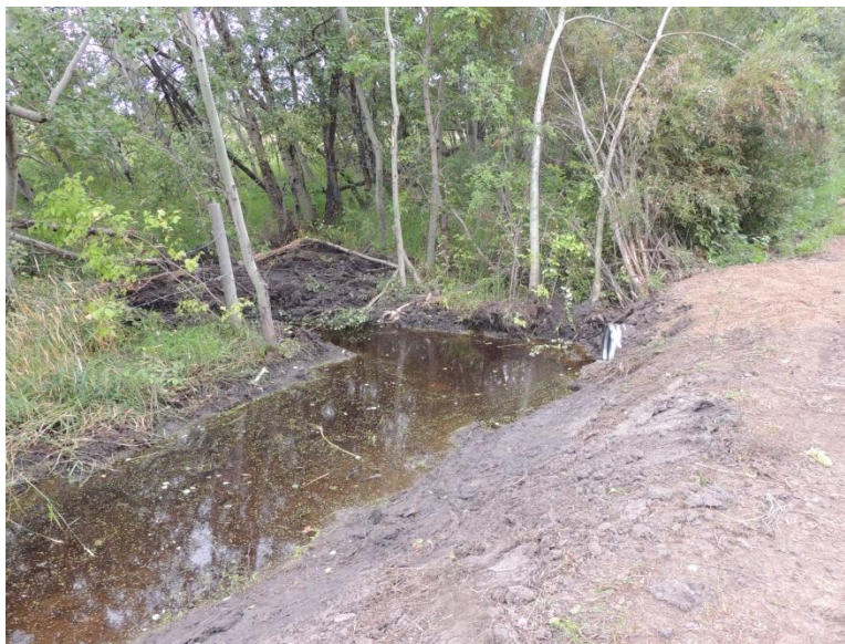
Figure 10: Newly installed culvert near 503 9 th Ave E
