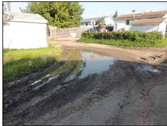
Figure 21: Alley between Cochin Ave and 6 th Ave W
