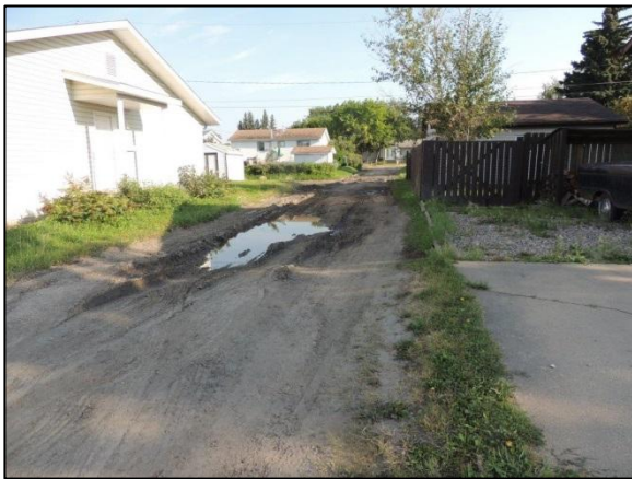
Figure 20: Alley between Cochin Ave and 6 th Ave W
