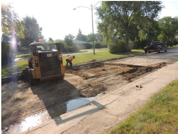
Figure 7: Pavement works on Centre St
