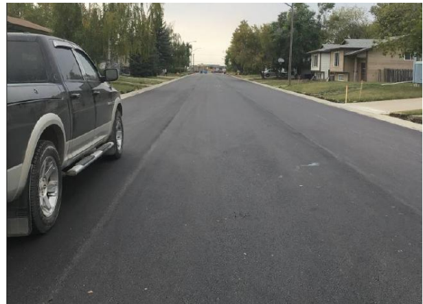
Figure 2: Cochin Ave after construction
