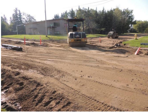
Figure 5: Base preparation on 6 th Ave W and 3 rd St W
