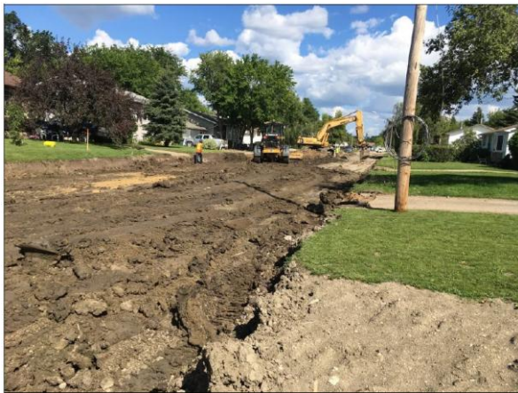
Figure 1: Cochin Ave during excavation for road construction
