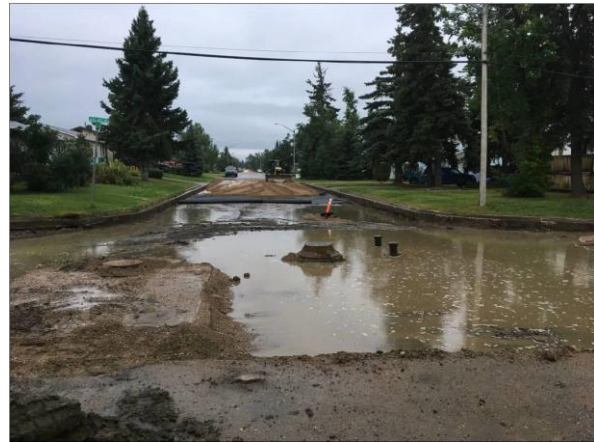
Figure 4: Intersection of 6 th Ave W and 2 nd St W before construction
