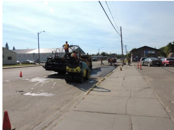
Figure 8: Pavement works on 2 nd Ave W and 1 st St W intersection
