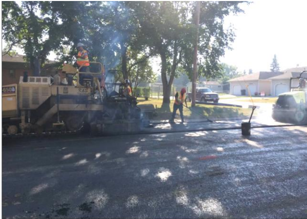
Figure 3: Paving on 4 th St W
