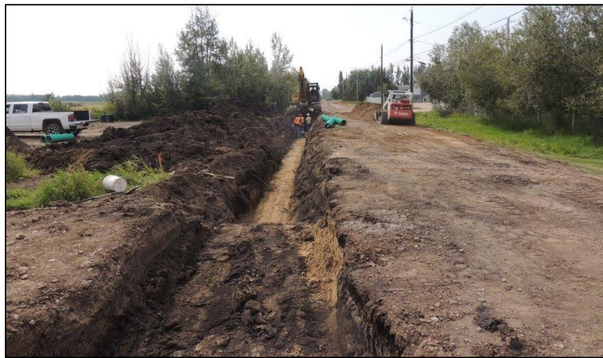
Figure : Storm pipe installation by Tupper Construction
