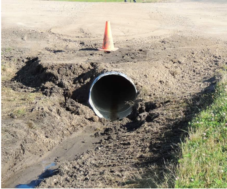
Figure 9: Newly installed culvert between 9 th St W and Highway # 4
