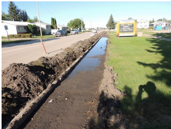
Figure 18: Sidewalk installation work near Gateway Elementary School
