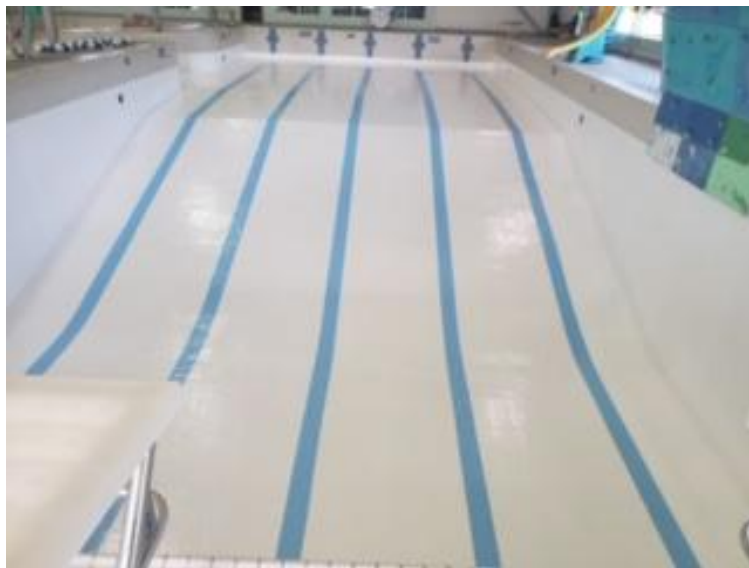
Repainted pool basin
